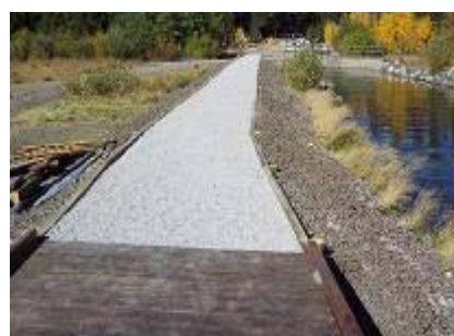
Accessible path to pier
